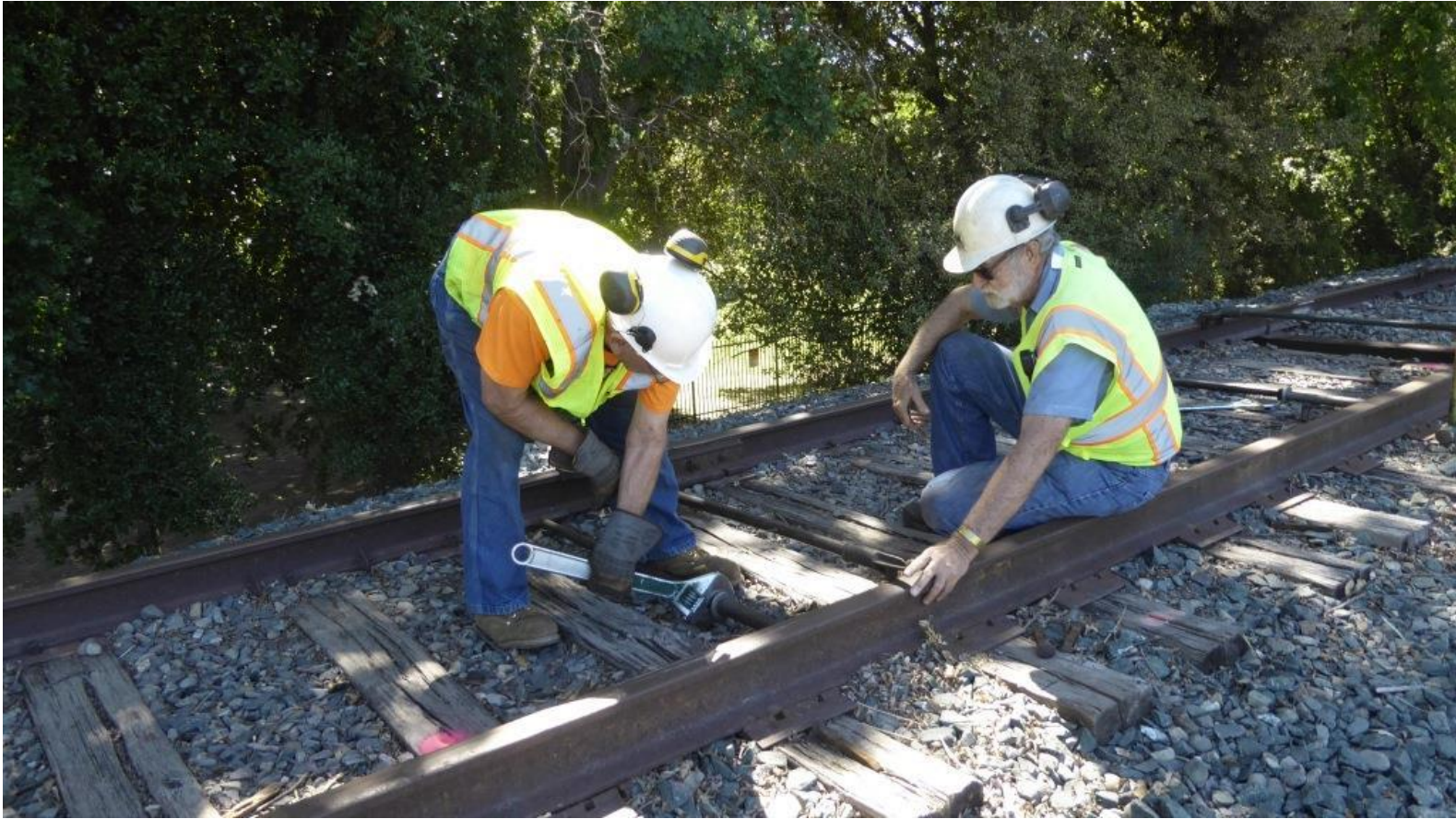
Clem spreads the rails with the rail-spreader as Alan monitors the track-gauge
