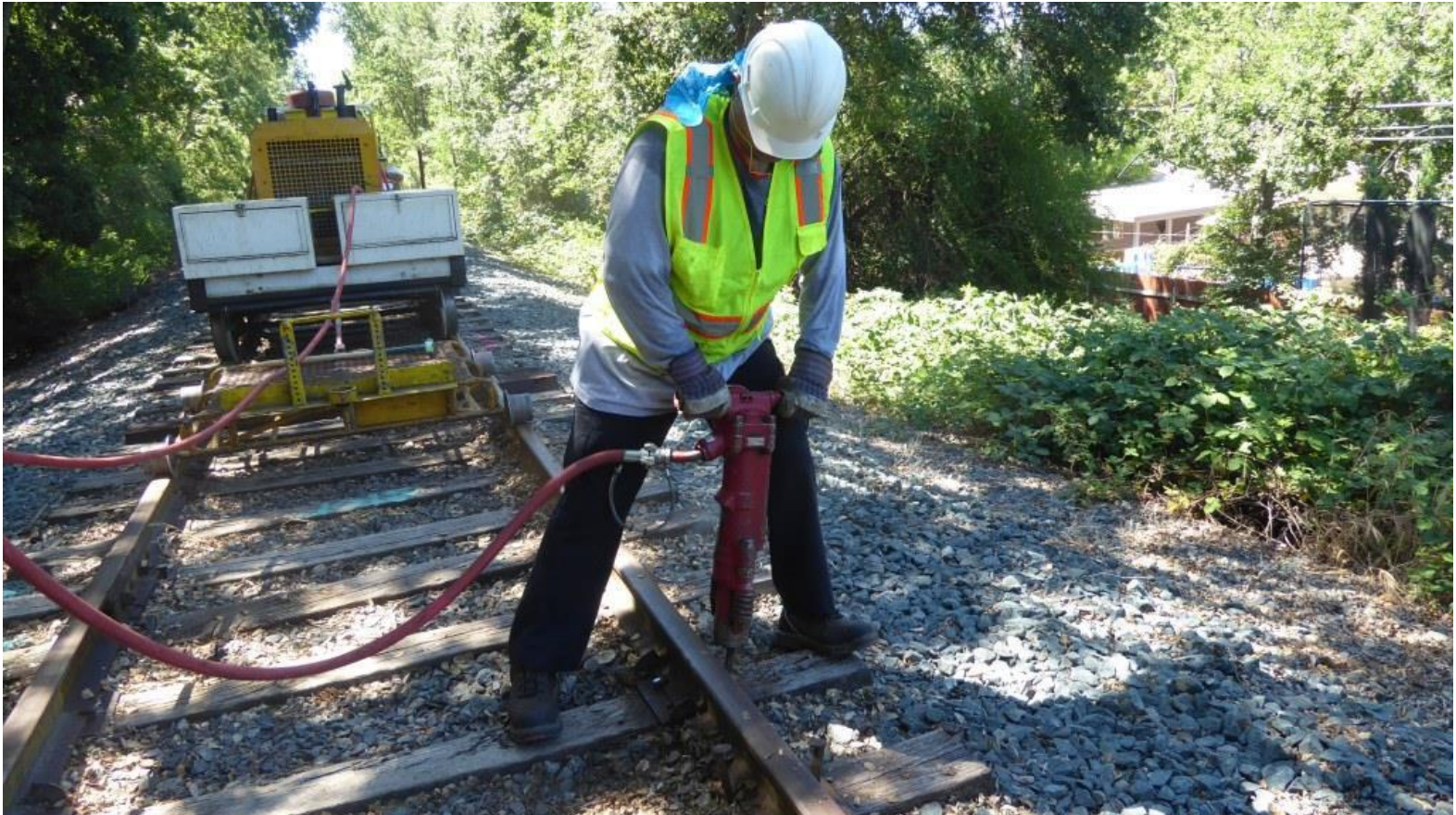
Jose drives spikes with the pneumatic spike-driver
