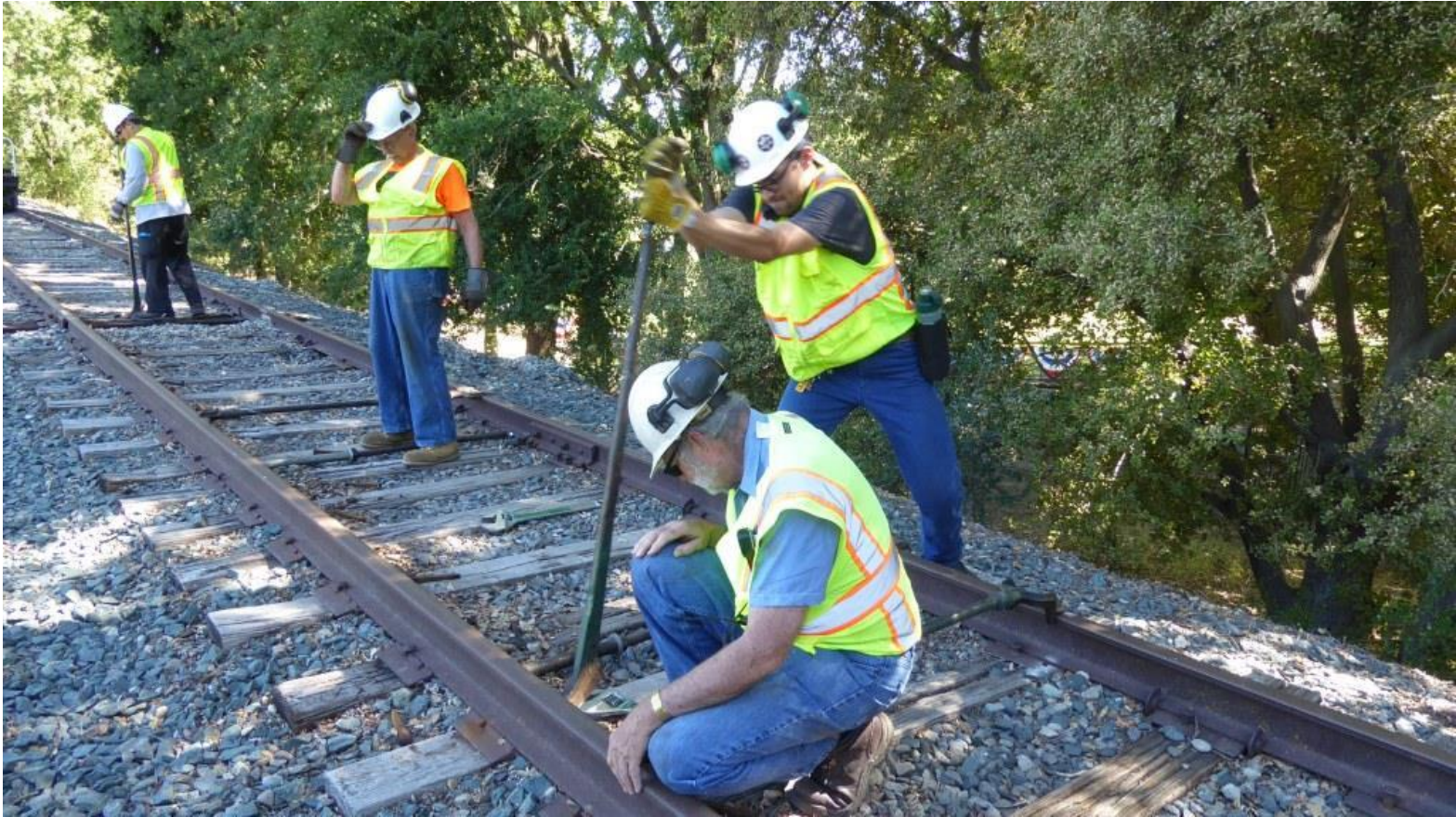
Kyle removes spikes in a narrow area so that the track can be spread
