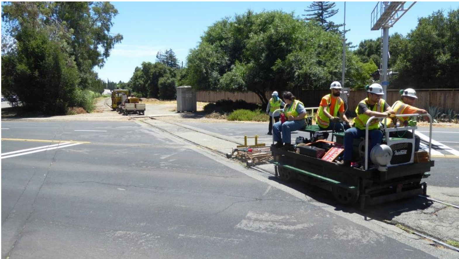
After lunch, the Team crosses Sutterville Road and heads back to the job-site
