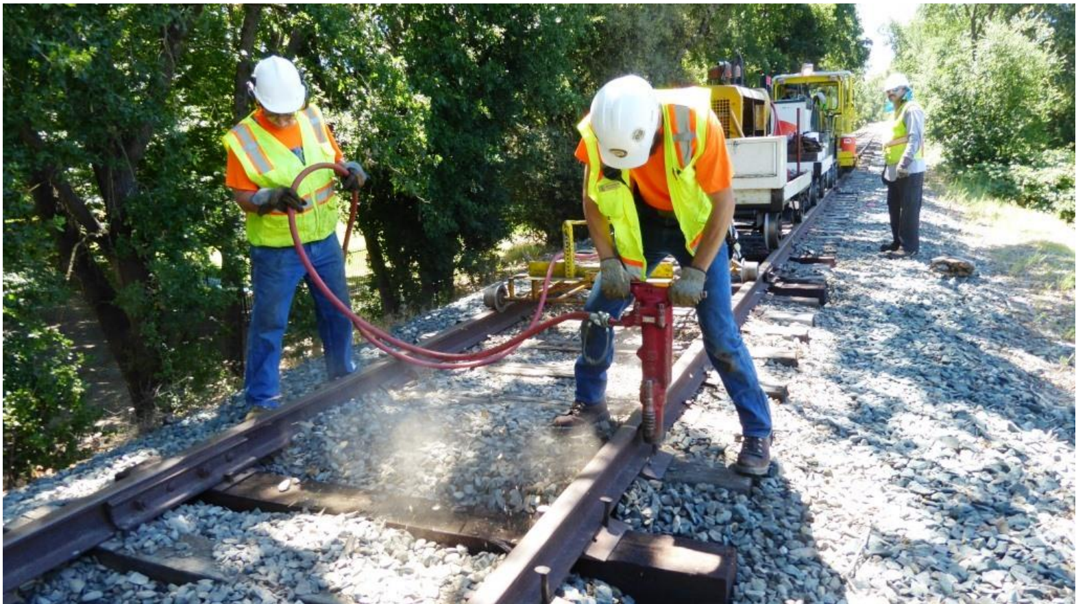
Now Matt takes a turn using the pneumatic spike-driver
