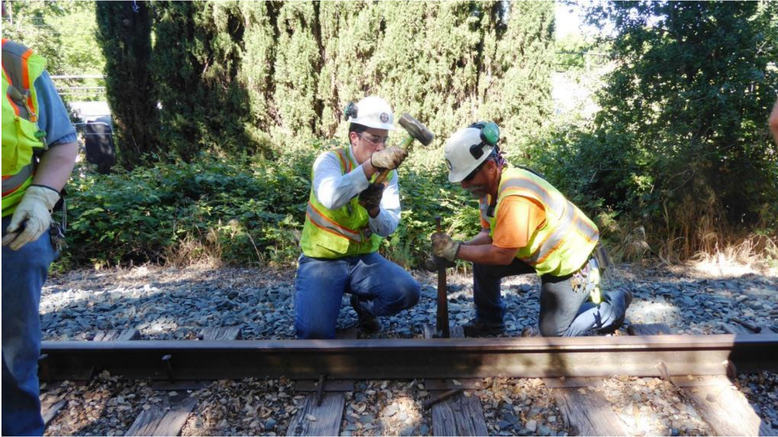
The hammer-head was loose so Weston and Joe drive a wedge into the handle to tighten it up
