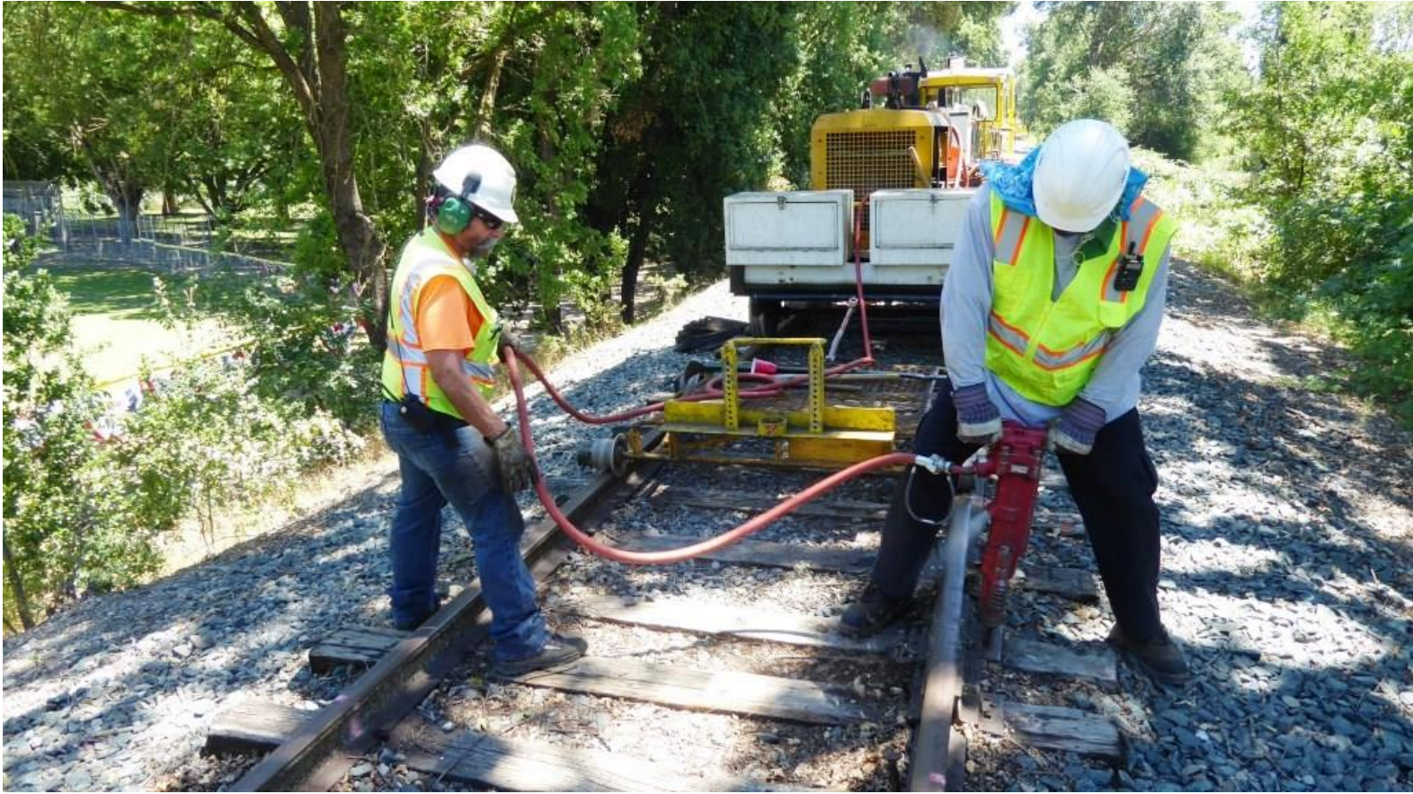
Joe guides the air-hose as Jose drive spikes
