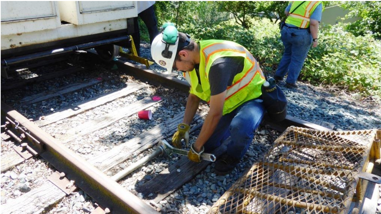
Kyle removes the rail-spreader
