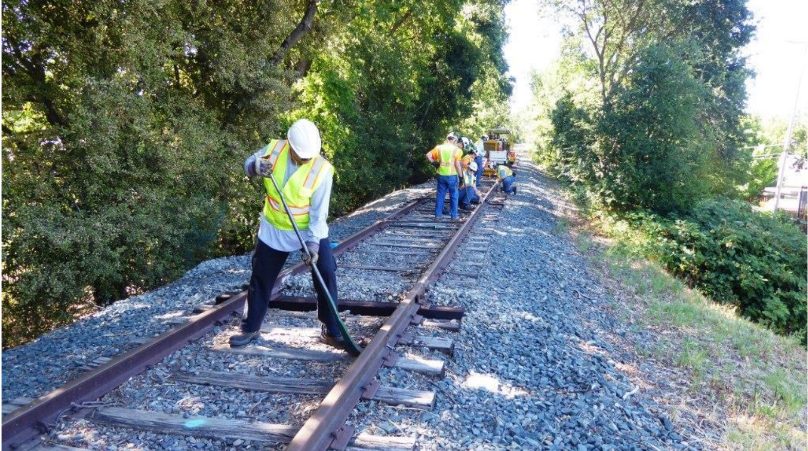
Further up the line, Jose keeps on pulling spikes
