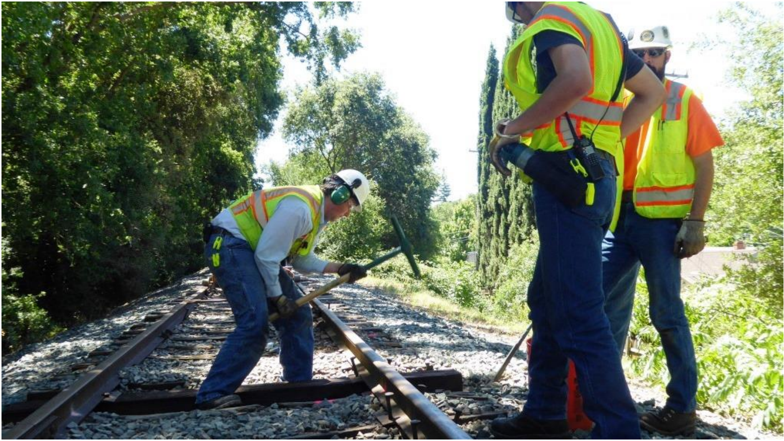
Spiking has caught up with the gauging so, Weston decides to drive a spike the old fashioned way
